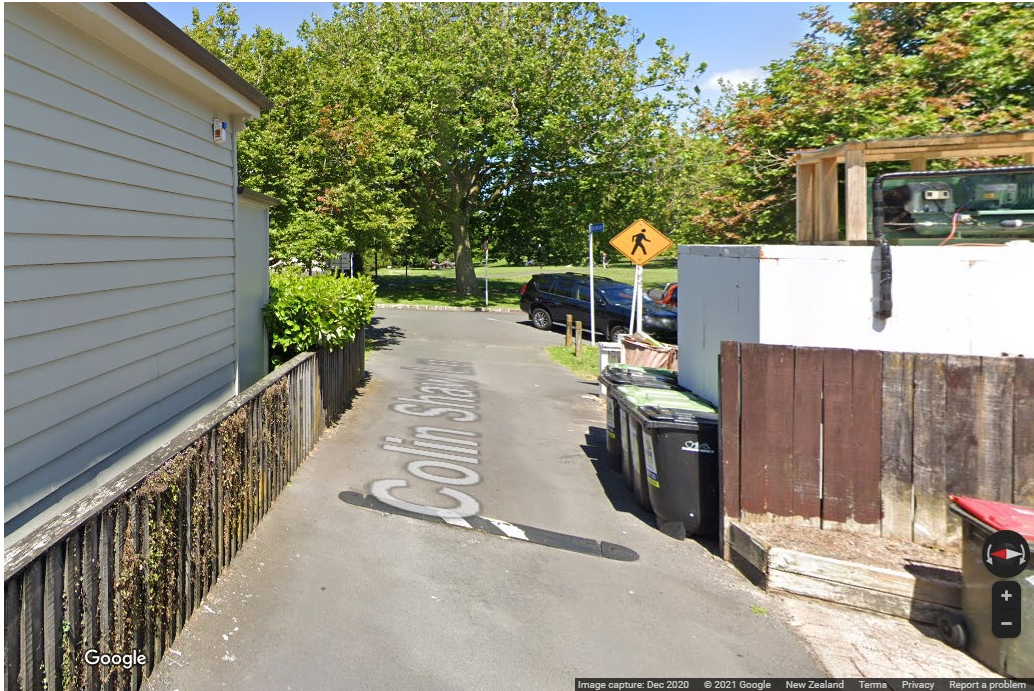
Figure 3: The existing exit point from the service lane at 2 Hepburn Street. Note the hedge on the left which has the potential to obscure visibility of pedestrians.
